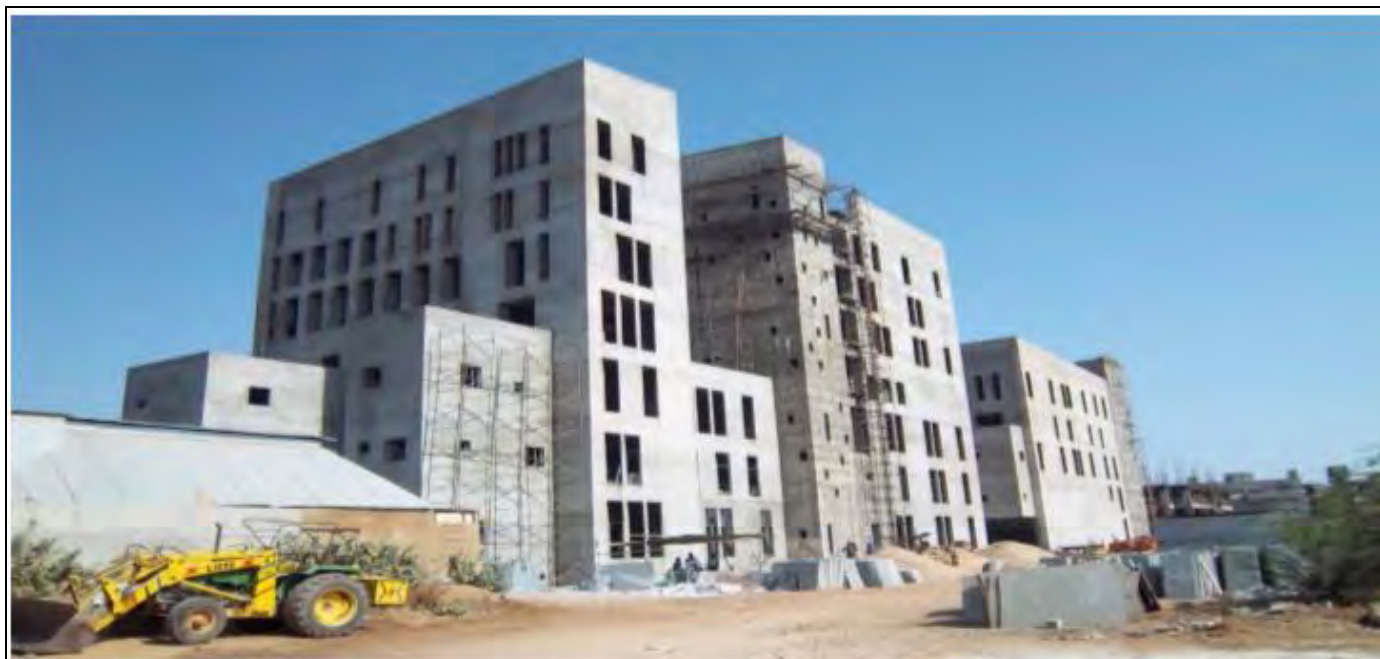
Fig. 1: INFLIBNET Centre's Building under Construction
